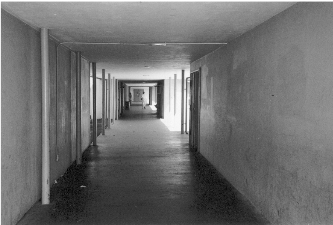
Figure 7: Covered walkway supported on pipe columns
