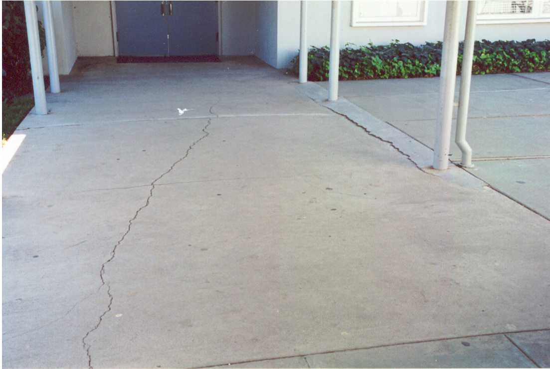
Figure 8: Cracks in existing slab-on-grade
