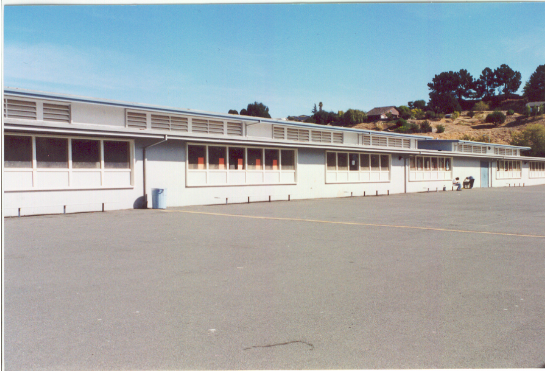
Figure 6: Exterior longitudinal (rear) wall of classrooms ( No.'s 19 to 22) with clerestory windows.
