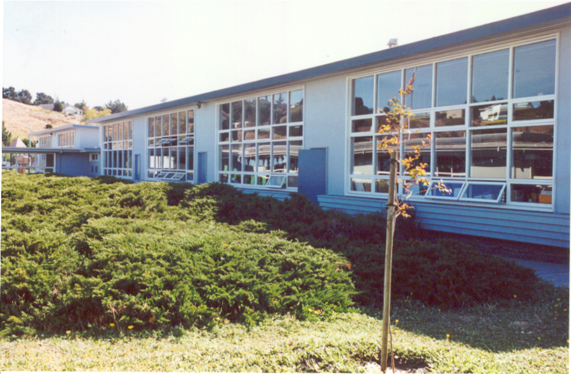
Figure 3: Exterior (front) wall of Classrooms 19 through 22
