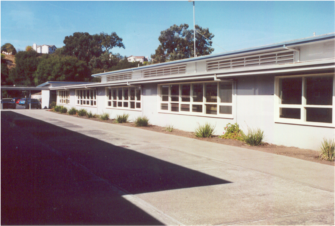
Figure 5: Exterior longitudinal (back) wall of class rooms with clerestory windows
