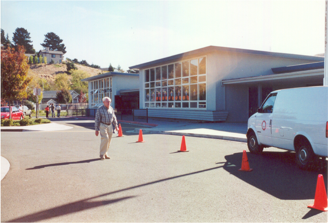
Figure 4: Exterior (front ) wall of Kindergarten classroom
